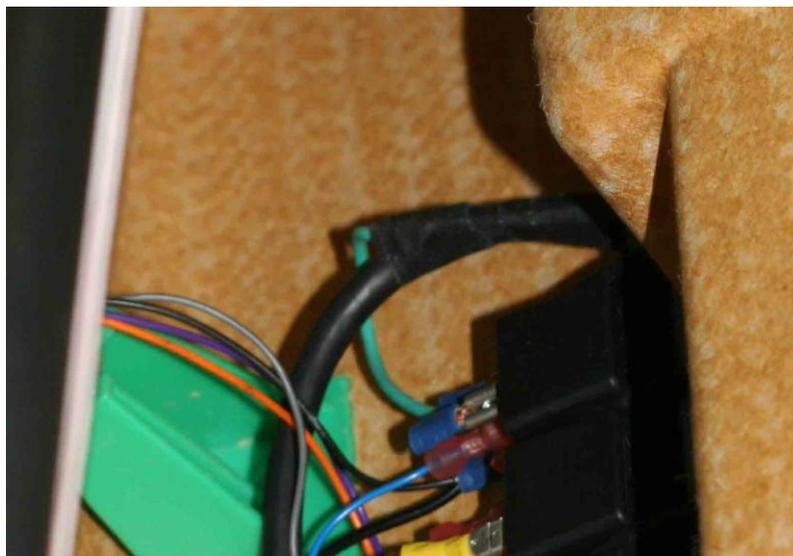
**Step 37:** Crimp blue quick connects on the green and white wires. Connect the green wire to Relay 3, terminal 30. Connect the white to wire Relay 3 terminal 86. The black wire is not used and can be trimmed back to the cable jacket.
